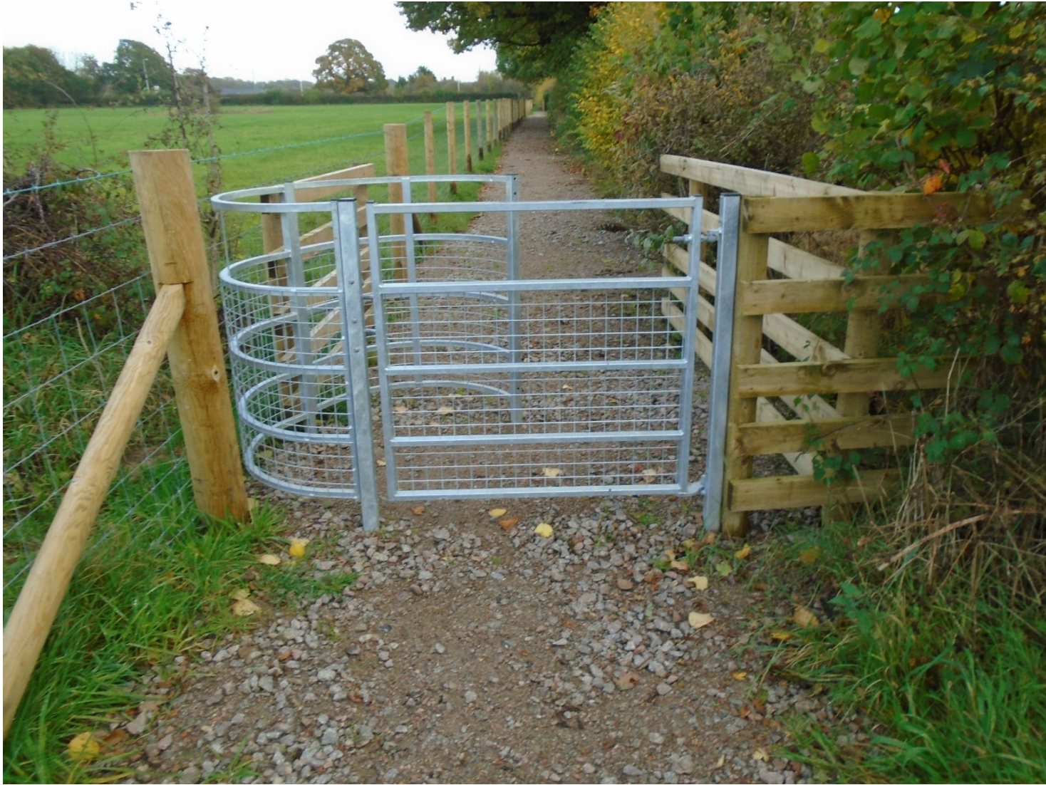
Another new gate – and improved path surface.
