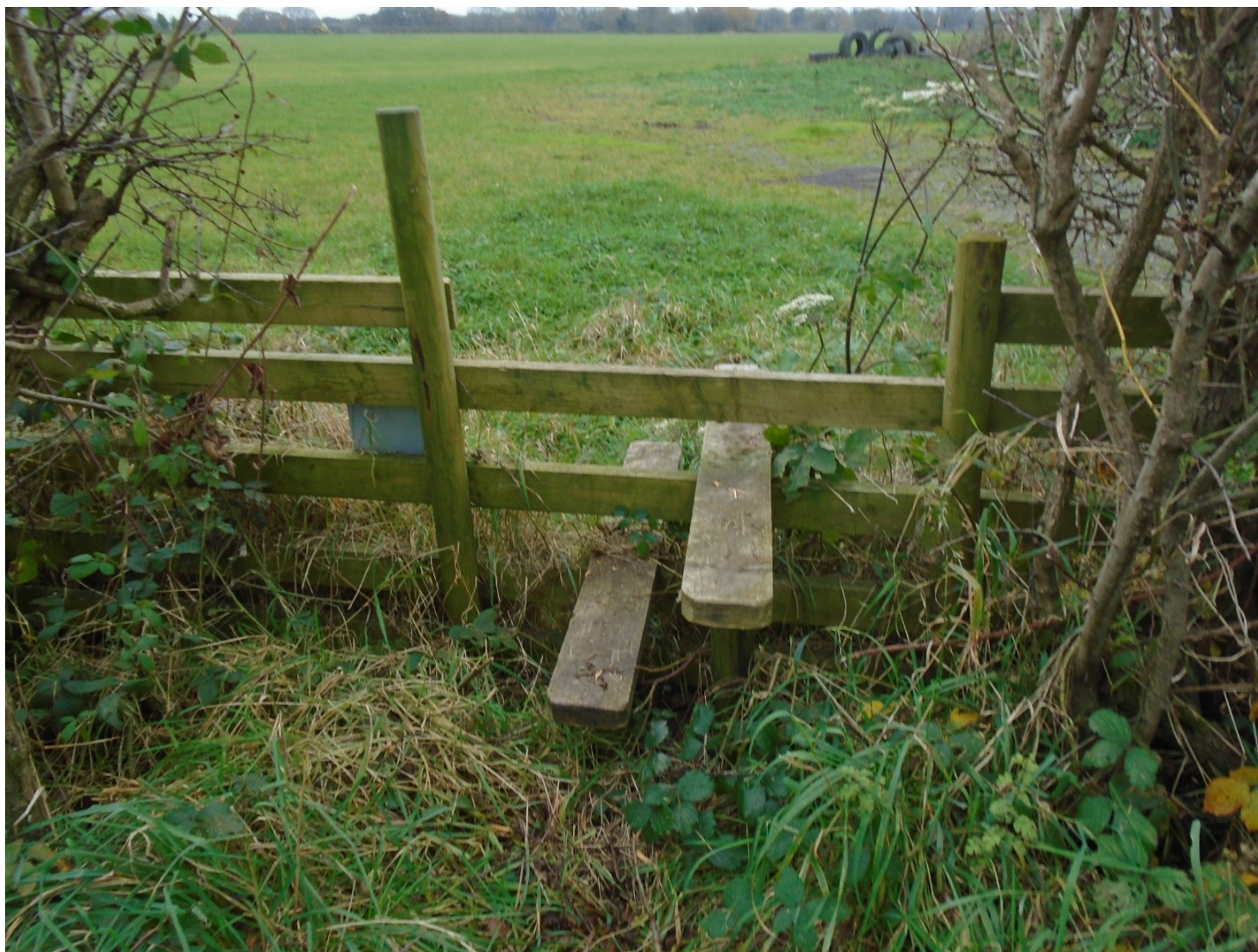
A stile repaired.
