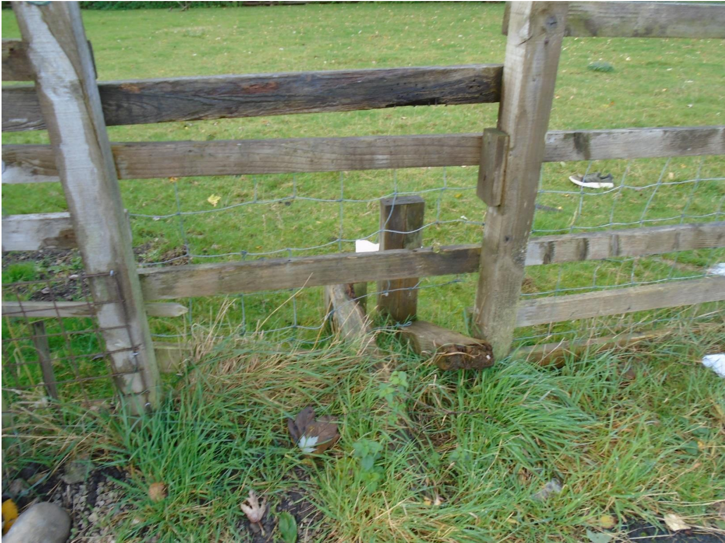
A broken stile.
