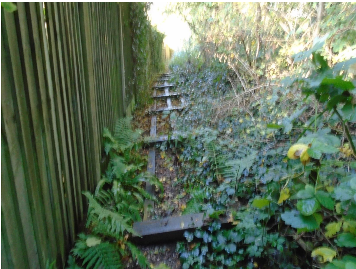
Broken fence having fallen onto the footpath.
