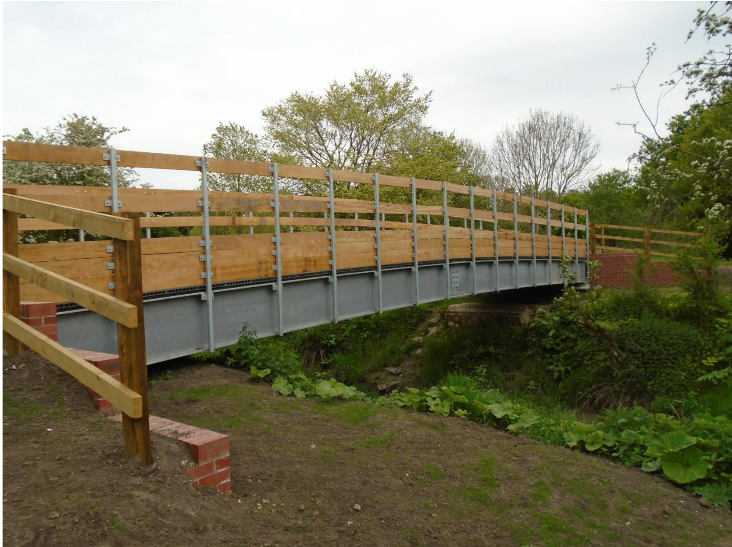
Another view of the replacement footbridge.
