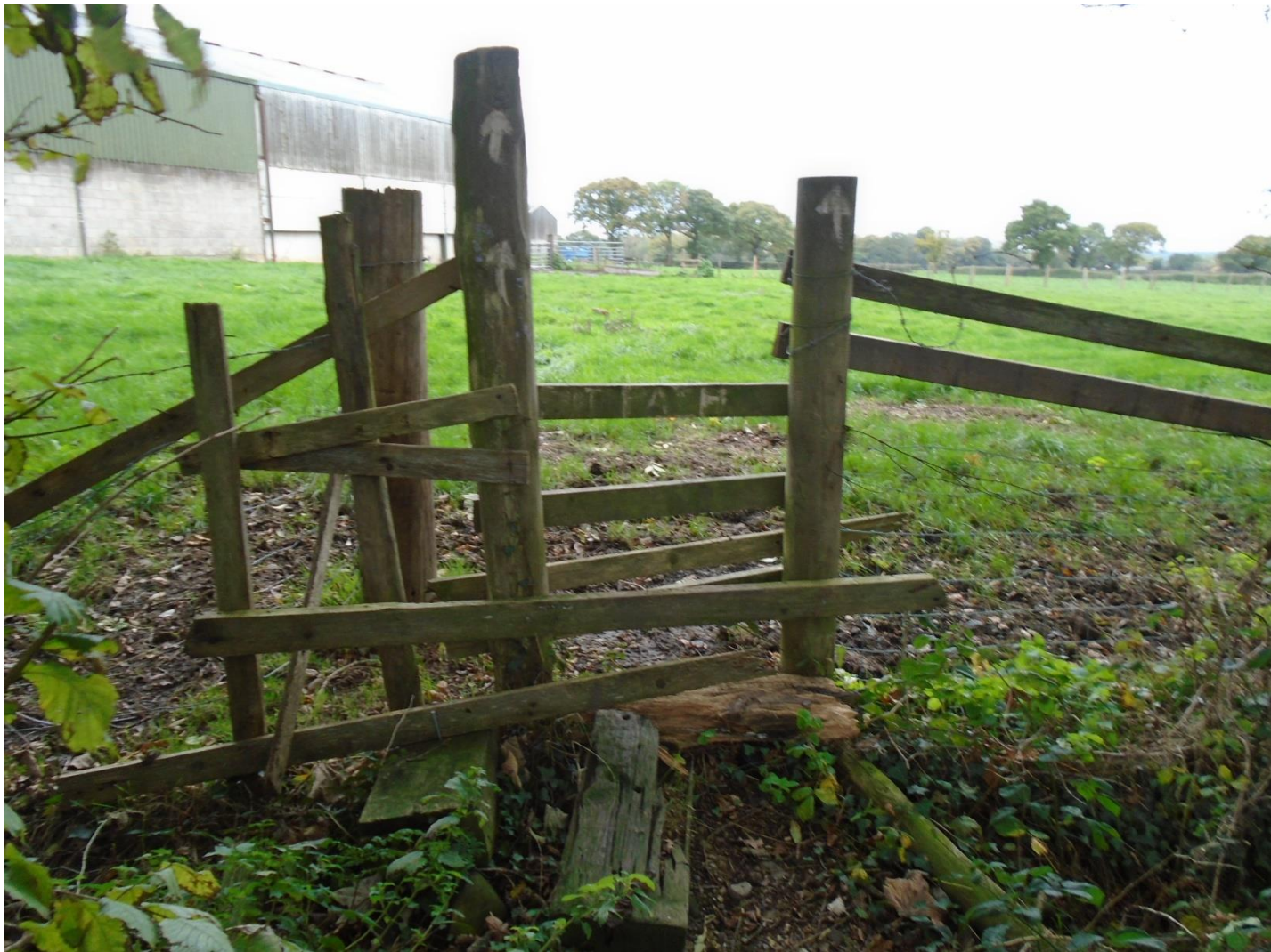
And another broken stile.
