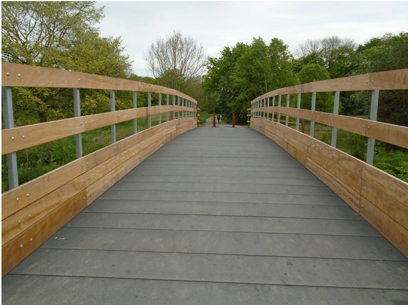
A replacement footbridge over a small tributary of the River Ribble – east of Penwortham.
