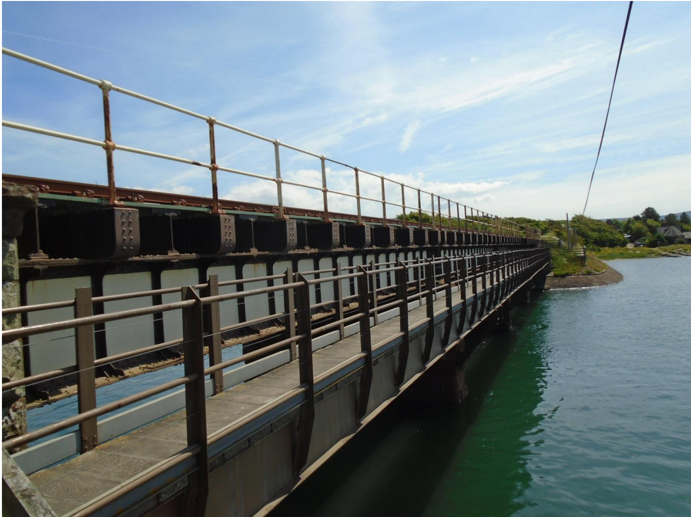
A footway bolted to side of the railway bridge over the River Mite at Ravenglass.
