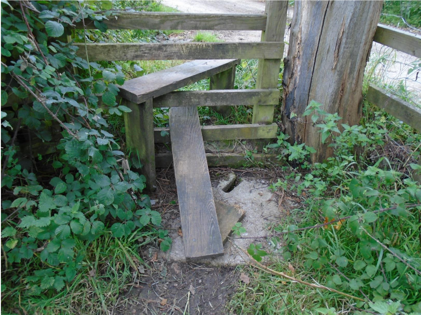
And another broken stile.
