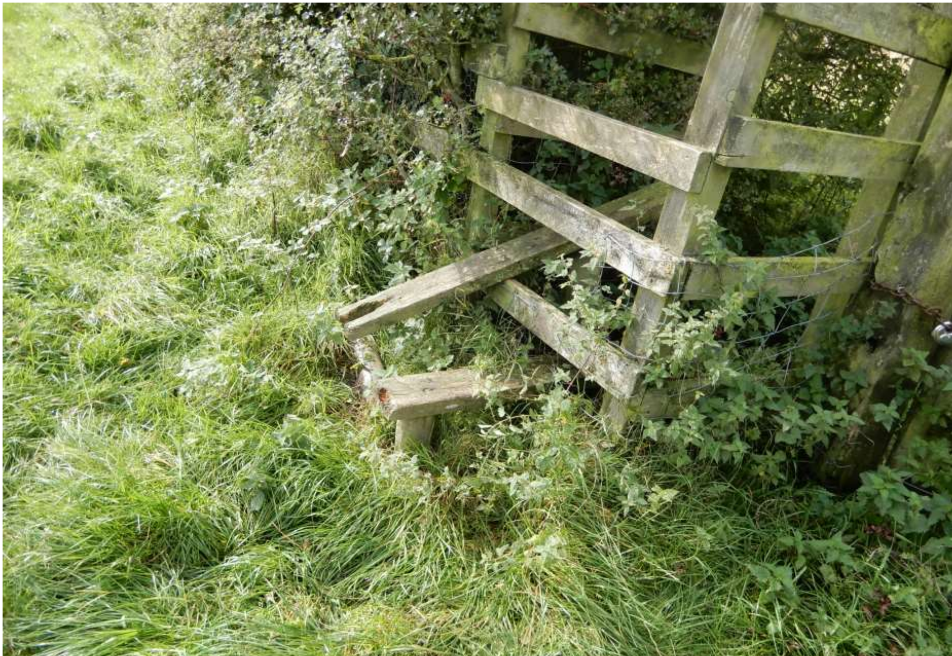
Another broken stile.
