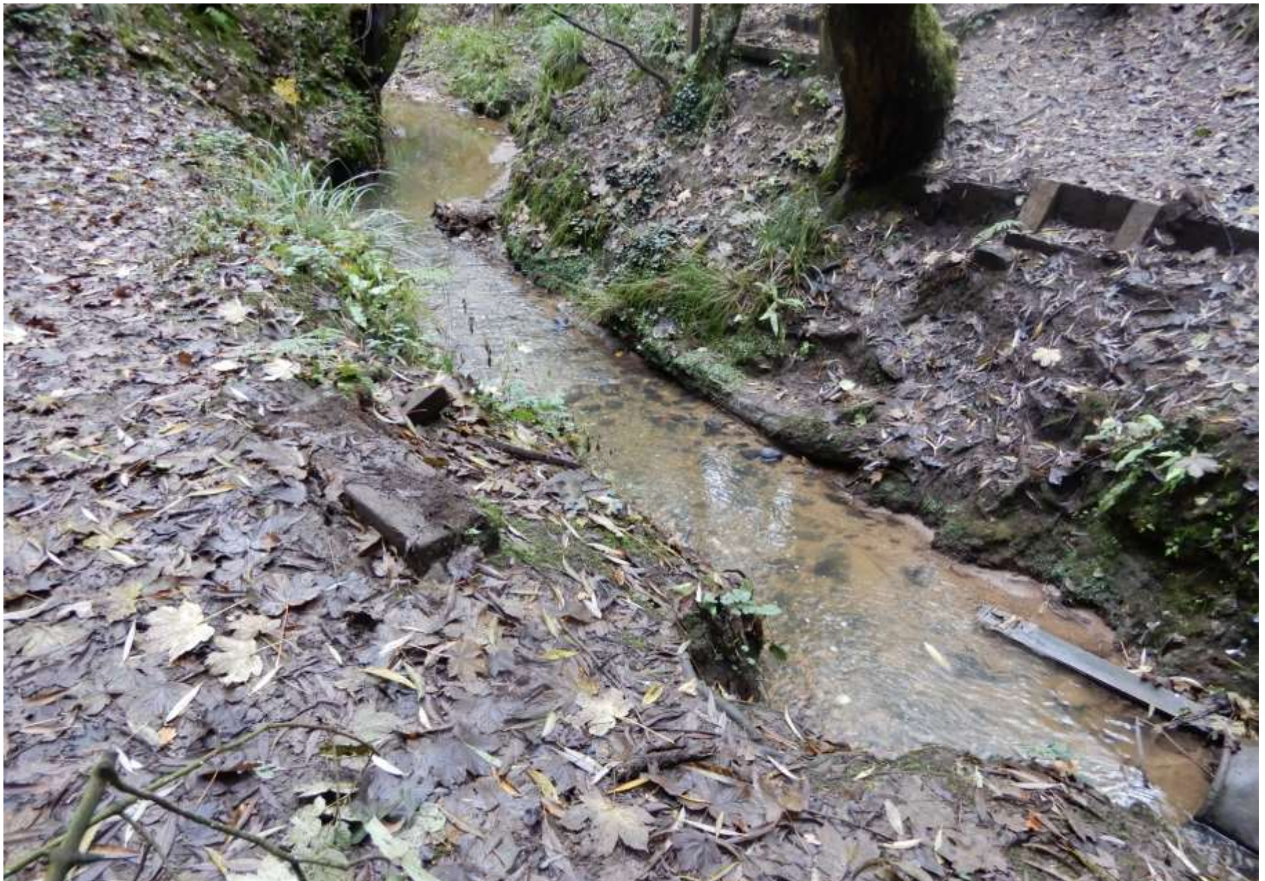
A footbridge that was lost in the floods.
